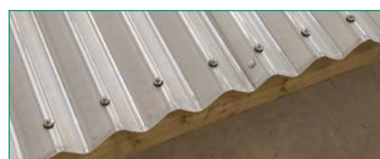
1 Primary Fixing At every corrugation
