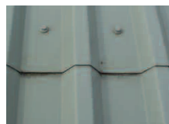
Colorcoat HPS200 with Galvalloy® roof after 7 years.
